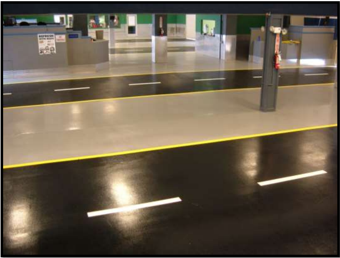
Manheim Phoenix, 21,000 SF Thin-Film System | Phoenix, AZ
