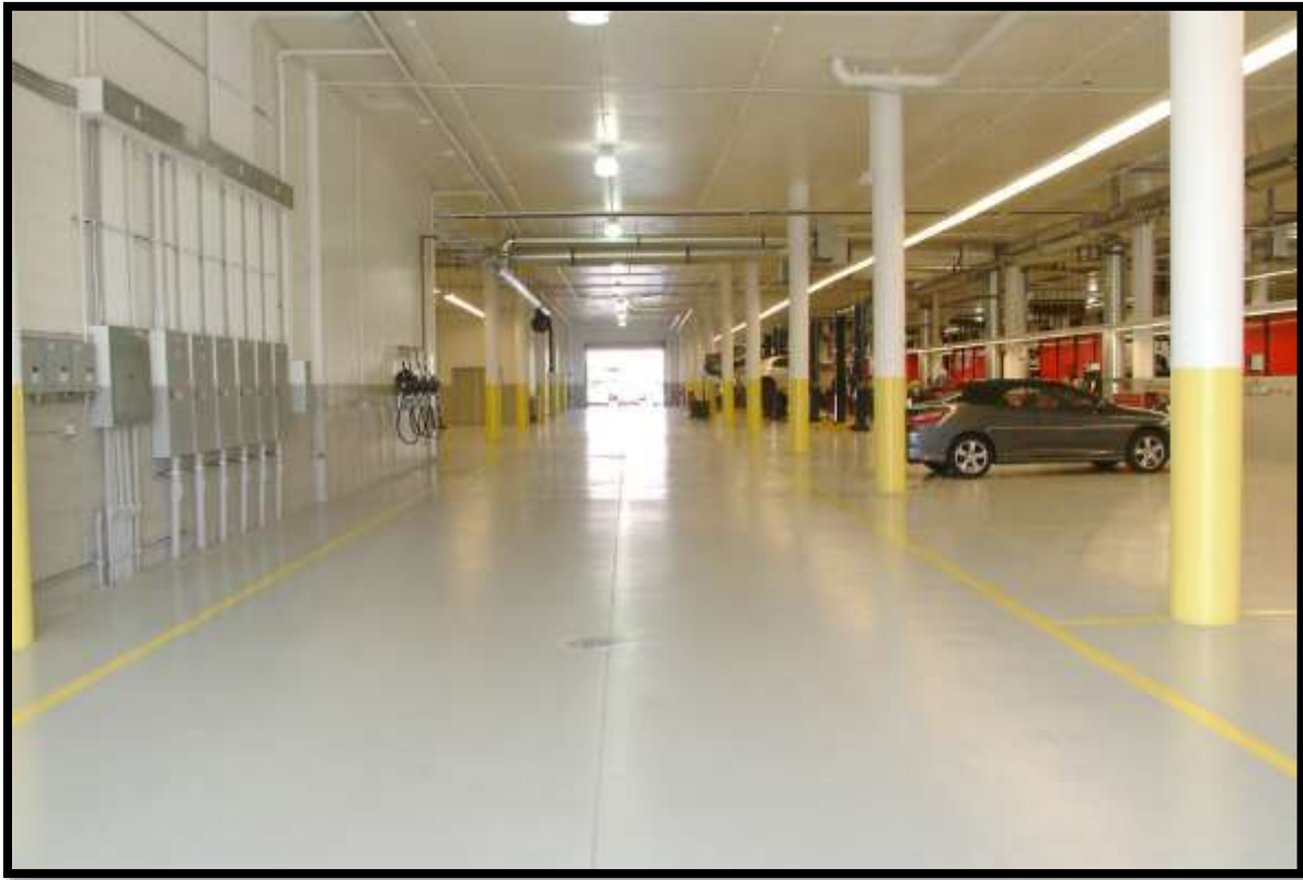
Carson Toyota, 38,000 SF Diamond-Epoxy Mortar Overlay | Carson, CA
