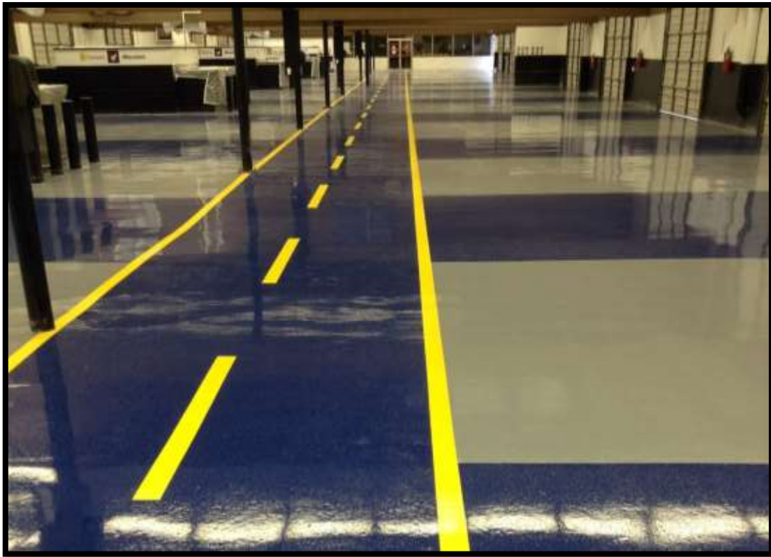
Manheim Houston , 21,000 SF Diamond-VRS Unlimited Moisture Control System | Houston, TX
