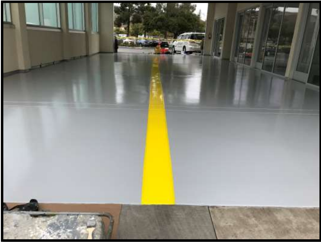
Infiniti of Thousand Oaks, 1,700 SF Diamond-VRS Unlimited Moisture Control | Thousand Oaks, CA
